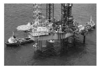
Figure 2 — General view of the offshore oil platform, which used steel piles with aluminum coatings
